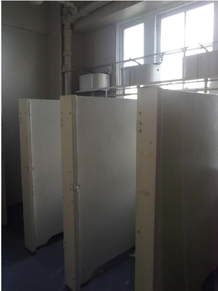
Figure 56: Amenities on ground floor of AML&F building display timber partitions and elevated cisterns. Level 3 amenities have terrazzo partitions which were likely to be an upgrade for the level that wool buyers would have frequented. Low level cisterns which extant on level 3 were probably installed in the 1980s.
