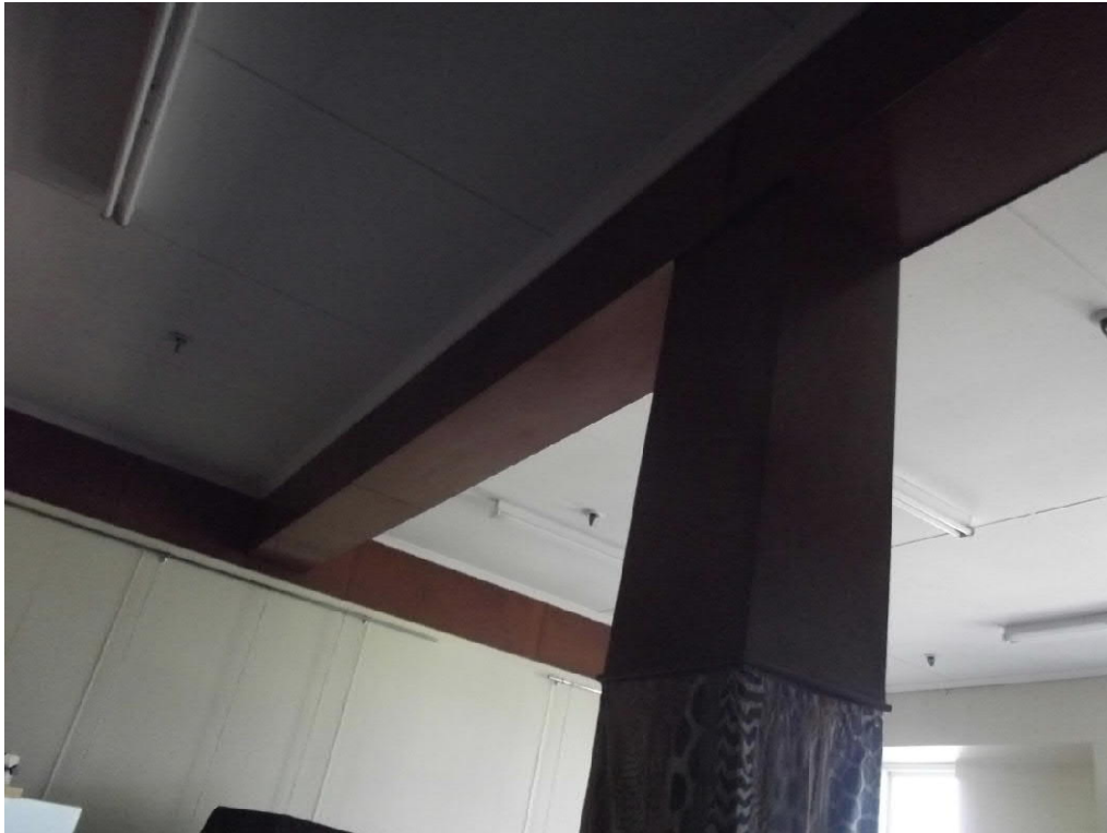
Figure 45: One of the rare ceilings in the AML&F building in the offices on the third floor. Ceiling appears to be lined with expressed jointed fibre cement. The Bearer and columns have been boxed in and lined with timber panelling.
