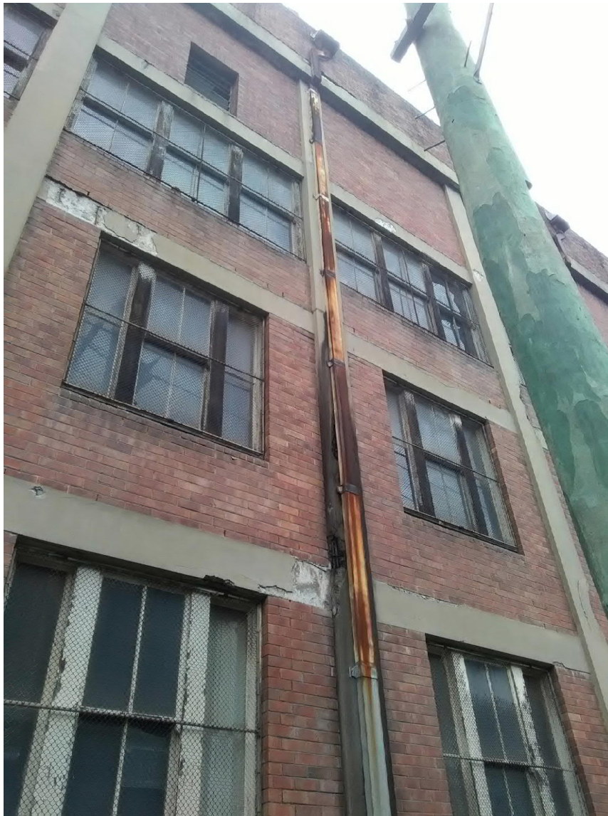
Figure 47: West facade of AML&F building showing rusted rainwater head and downpipe with offset and water staining on the concrete column caused by water escaping the downpipe.
