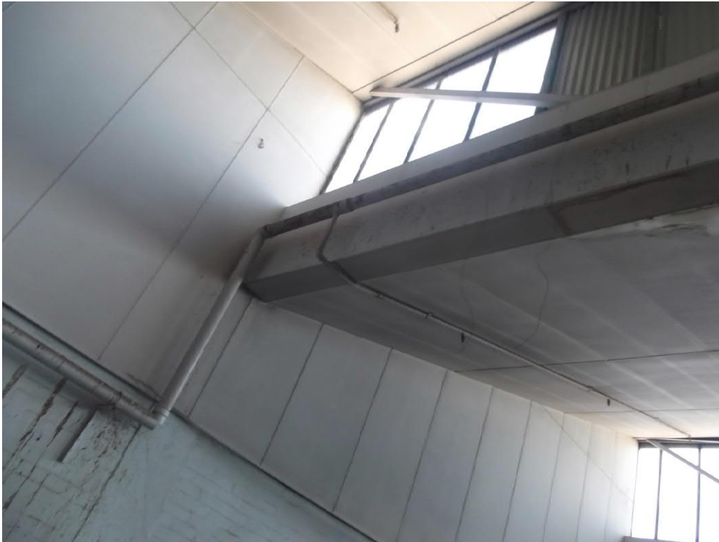
Figure 46: Small section of Sawtooth roof demonstrating internal linings, mixed infill to glazing frames, water leak damage to ceiling (centre right) and existing fire sprinkler services.
