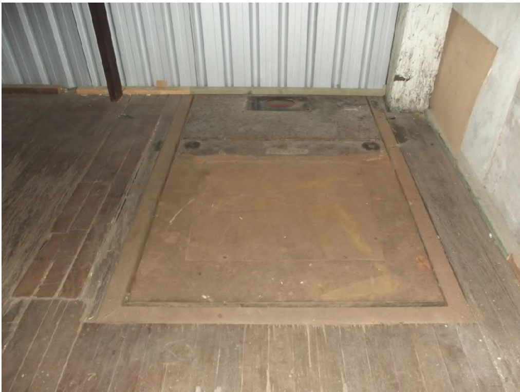
Figure 62: Trapdoors in the floor link between levels and to shafts demonstrate elements of the operation of the buildings.
