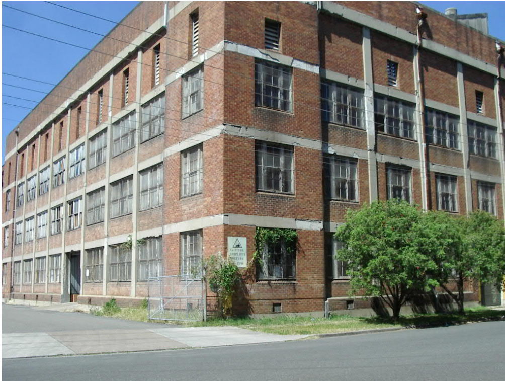
Figure 40: Window layout of AML&F building showing wider windows with spandrels on North side and third floor with narrower windows on corners and lower floors. Timber louvre vents on fourth floor.
