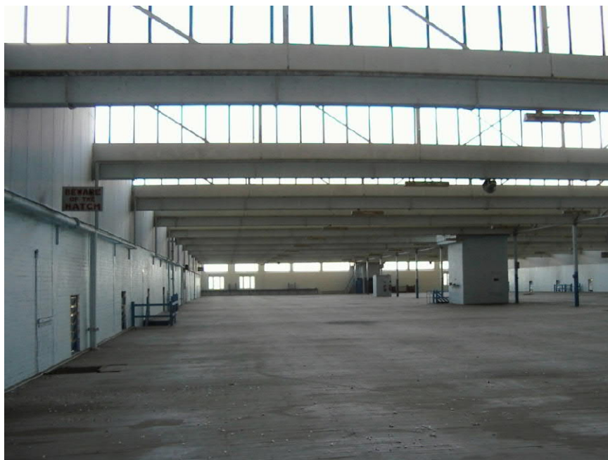
Figure 13: Typical Level 4 of AML&F Woolstore looking South with sky visible through the south lights. Abundant natural light is provided to the entire floor plate whilst avoiding direct sunlight. Note beside the south light glazing, the vertical and diagonal members of the trusses which support the sawtooth roof.
