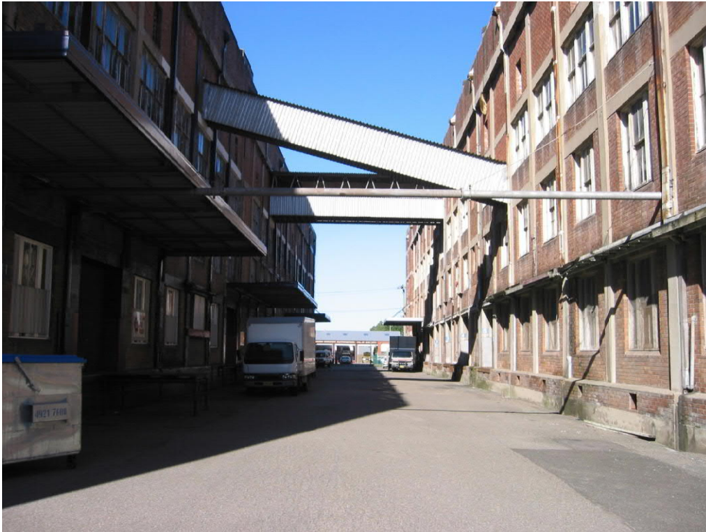
Figure 70: A wool bale chute and covered walkway link the AML&F wool store at right with the Dalgety wool store at left. An overhead water pipe which appears to be part of the fire sprinkler system is also evident.
