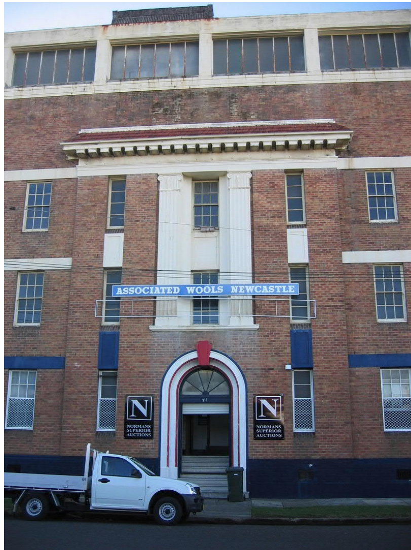
Figure 39: Annie Street Facade of NZLMA building displaying detail of pilasters, cornices dentils and friezes. Applied spandrel panels between the windows either side of the central door and the terracotta tiles over the entrance are unique to this building. There is a shadow of former NZL signage at the top of the building above the tiles.
