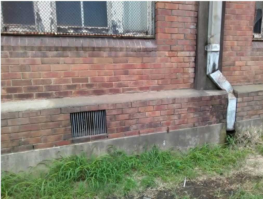
Figure 48: Base of same downpipe showing physical damage to downpipe as well as offset and constriction all contributing to water staining on the column. Downpipe does not appear to be connected to underground services, discharging onto the ground adjacent to the building's footings.
