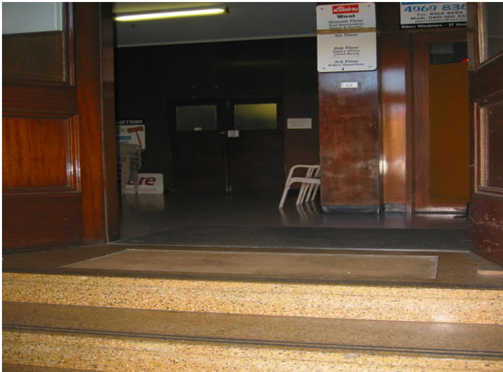
Figure 49: Main Entrance to the AML&F building, with timber panelling and vinyl floor covering. Note the terrazzo steps with integrated mat well.
