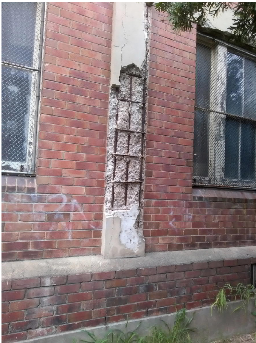
Figure 36: Some of the worst visible damage to the existing concrete structure, spalling on the West side of the AML&F building.
