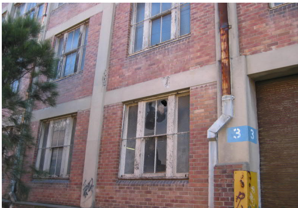
Figure 41: Western Facade of AML&F Building from Milford Street; note smashed windows, dry rot to sills, and rusted downpipes.
