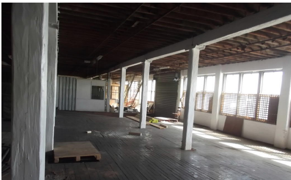
Figure 33: Ground Floor at Northern end of AML&F building shows uneven gaps, some cupping and warping from wear. Other areas have had sections cut out and replaced.
