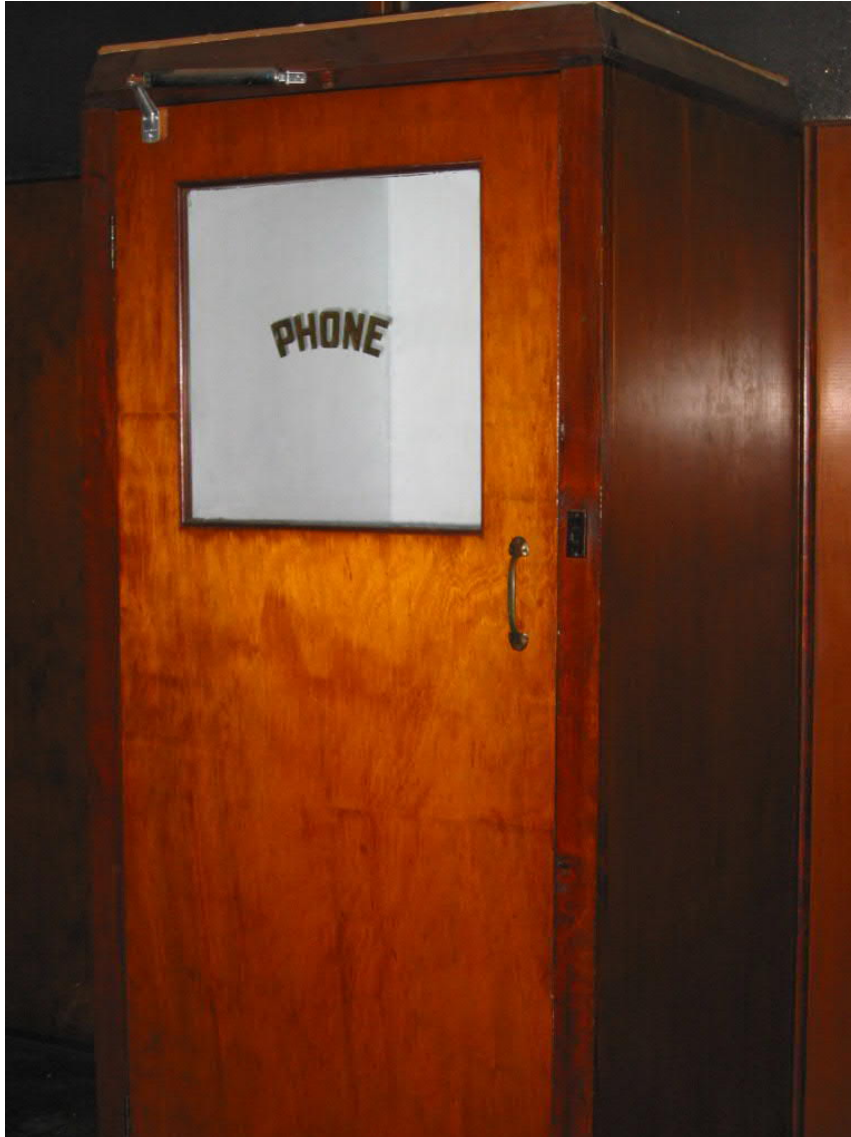
Figure 51: Joinery items such as the timber panelled public phone booth provided for wool buyers punctuate the public spaces of the buildings.
