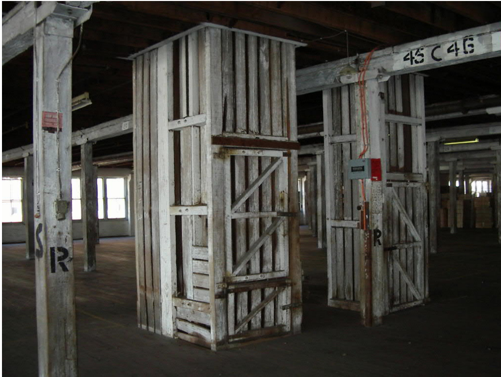
Figure 63: Wool Drops link most levels and demonstrate the operation of the buildings. They are constructed of heavy timbers with thick steel hinges and catches.
