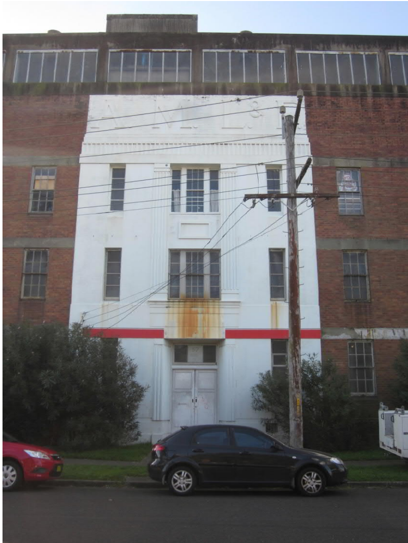
Figure 37: Annie Street Facade of AML&F building displaying detail of pilasters, cornices and friezes. Also visible is rust staining which washes down from the protective screens over the windows.
