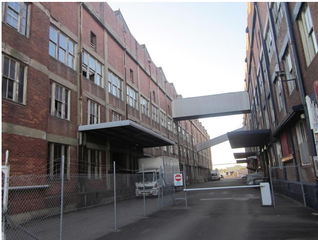
Figure 16: Driveway between AML&F and Dalgety looking north. Overhead walkway (horizontal) and wool chute (diagonal) are apparent. There is a horizontal water pipe between the two buildings just visible near the north end.
