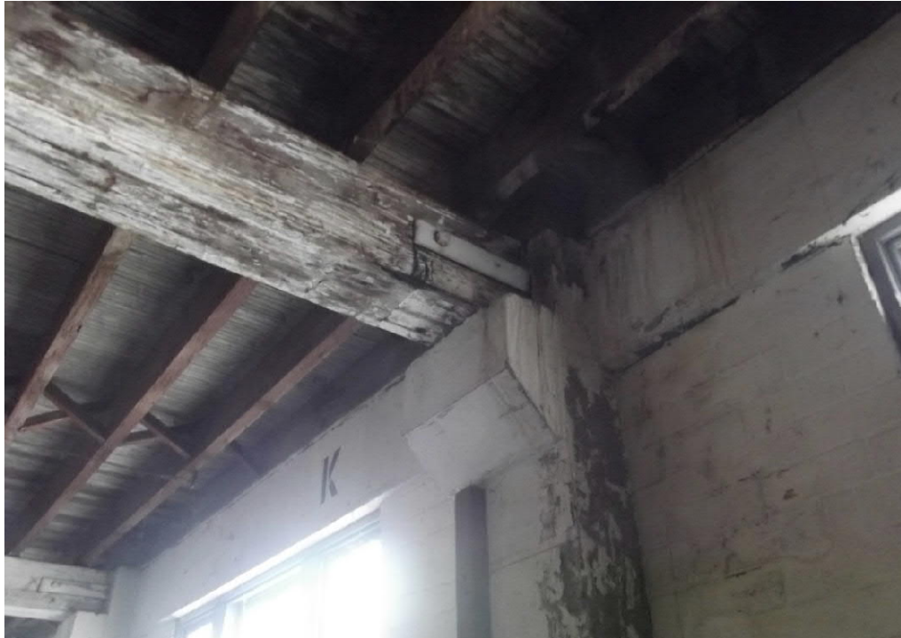
Figure 34: Bearer sitting on concrete corbel at external facade, paint finish deteriorated. Joists and herringbone blocking visible above left.
