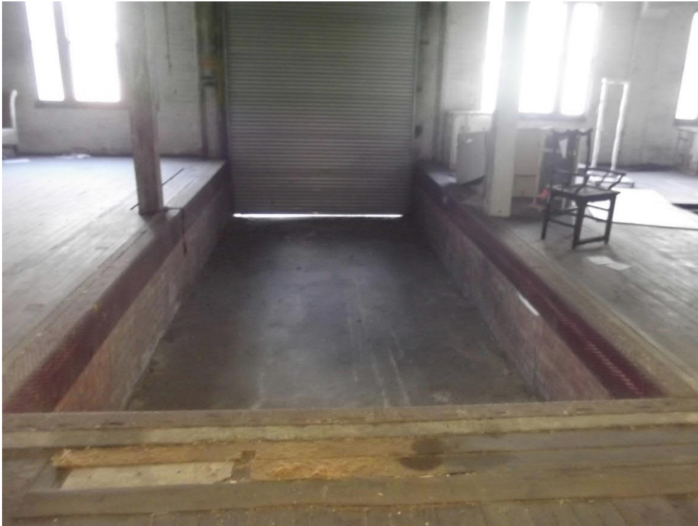
Figure 61: Loading Docks sunken below the floor level and fronted by roller doors demonstrate how wool bales arrived at and left the buildings. Some examples have been fitted with ramps up to the floor level.
