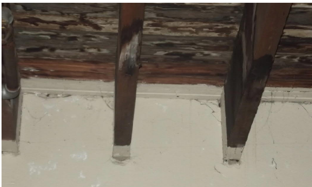
Figure 35: Floor joists (intersecting with an internal wall) water staining is visible on the floorboards and has extended to the joists also.
