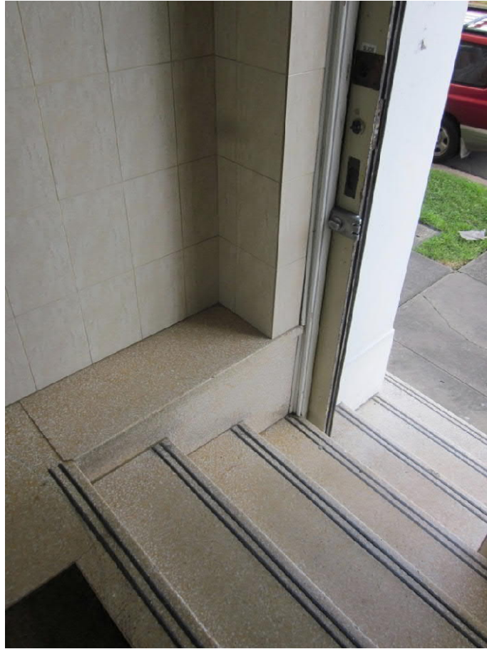
Figure 43: Inside the Annie Street Entrance door of one of the Woolstores. Note the main doors slide into the wall either side of the doorway.
